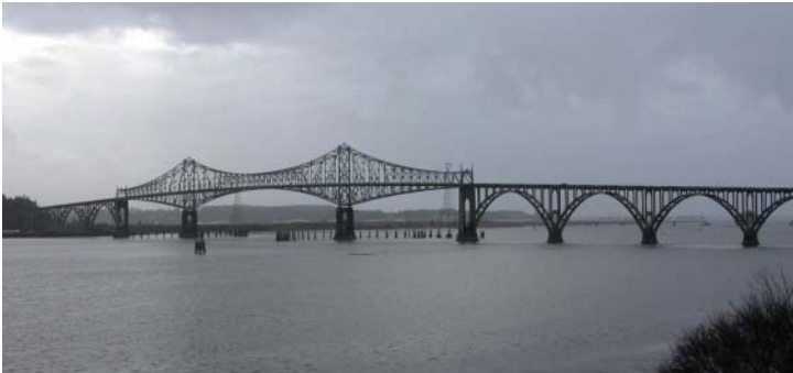
Conde B. McCullough Memorial Bridge
